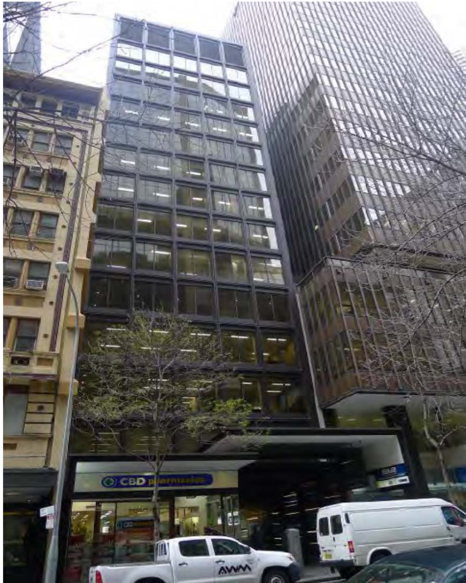
Figure 7 - Generally looking east from Pitt Street
