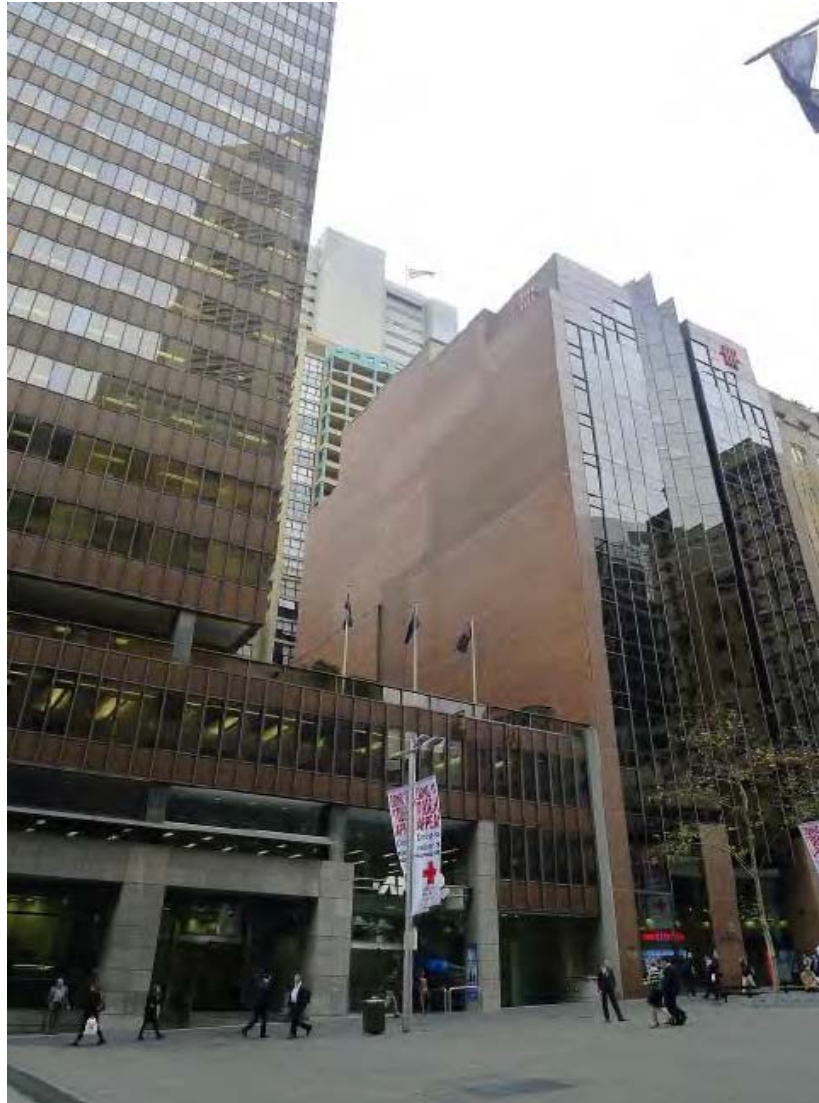
Figure 4 - Existing Martin Place ground plane
