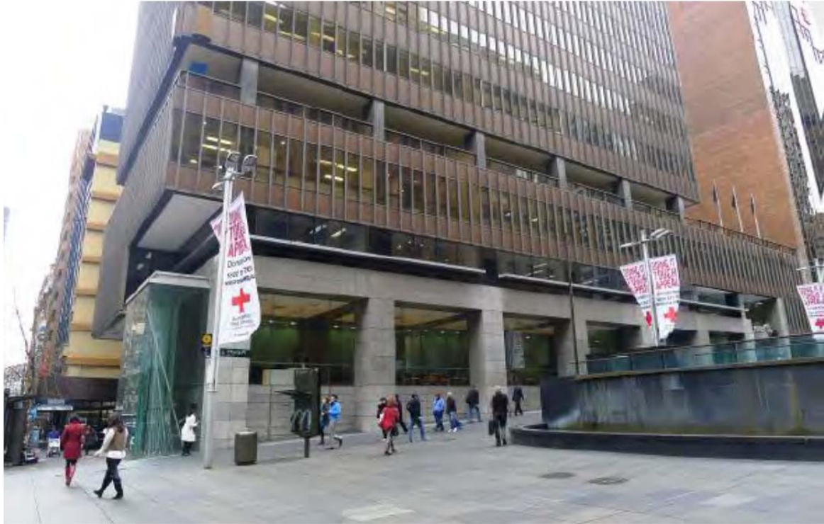
Figure 3 - Existing Martin Place ground plane
