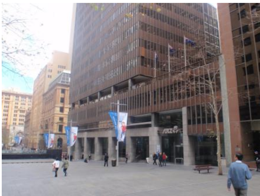
Figure 5 – Existing Martin Place ground plane
