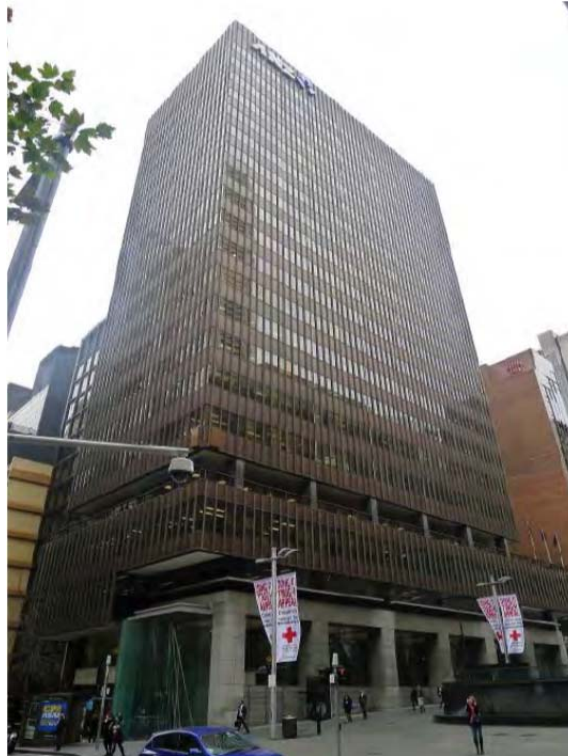
Figure 2 - View from corner Martin Place and Pitt Street
