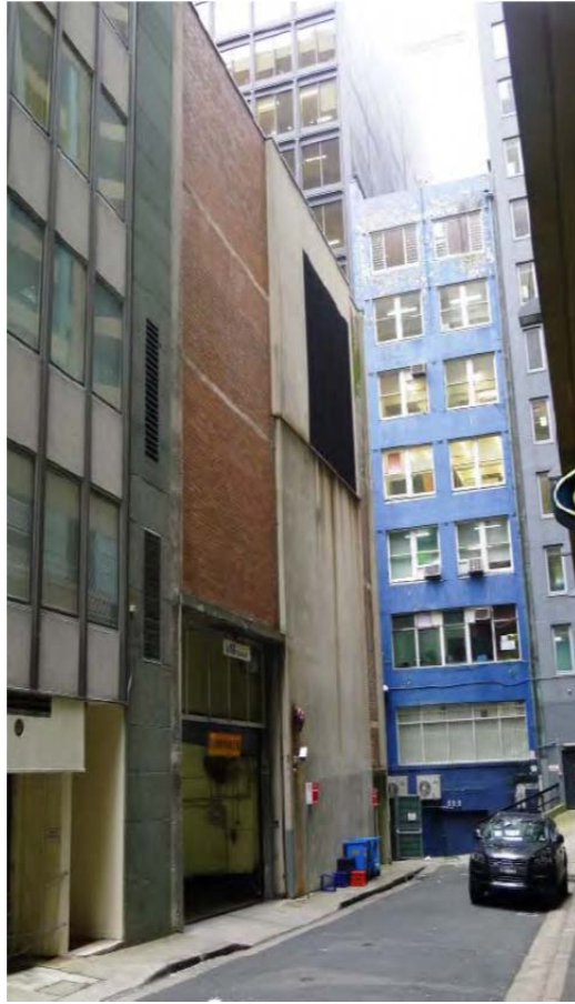
Figure 17 – Existing view of Hosking Place
